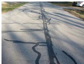
Since 2001 have been overlaying chip seal streets. One overlay does not give enough strength to be classified as hot mix
