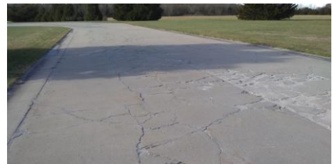
Burlingwood constructed in 1992 is only concrete street identified that has base or thickness issues.
